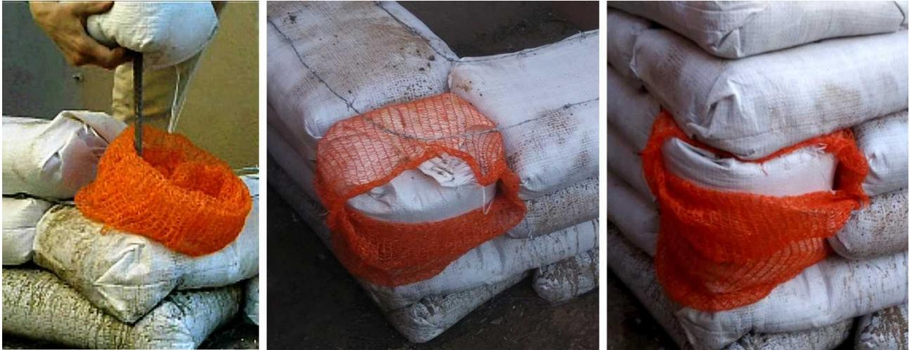
*Figure 33 A target sandbag for a covered splice (left to right): a- inserted over the rebar into a mesh tube; b- courses next to the sandbag; c- courses added to final wall height.*
