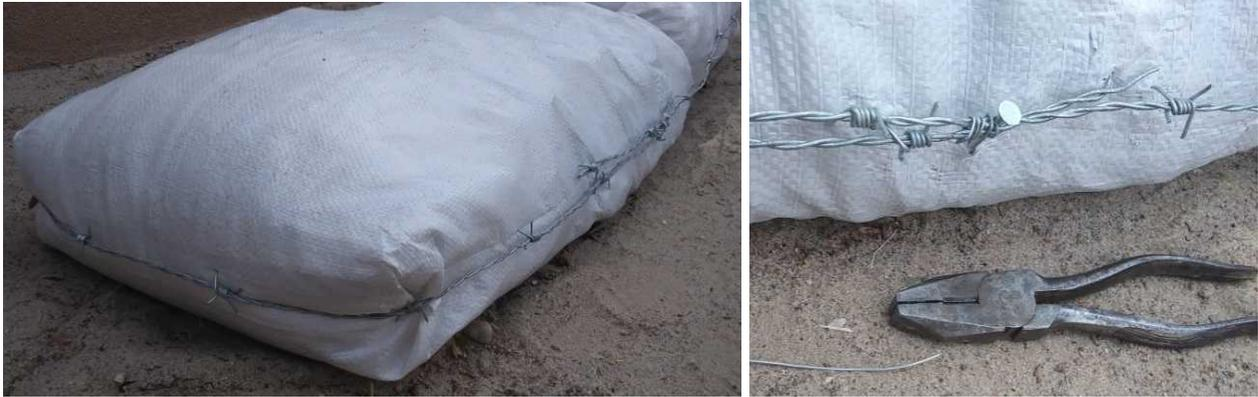
Figure 23 (left to right) Binding gravel bag courses: a- Wrap straight lengths; b- Attach securely.
