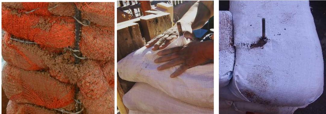
*Figure 25 Rebar in walls (left to right): a- must not be partially embedded in the edge of CE walls; b- can have bags punched onto steel; c- or tubes cut to form around steel.*
