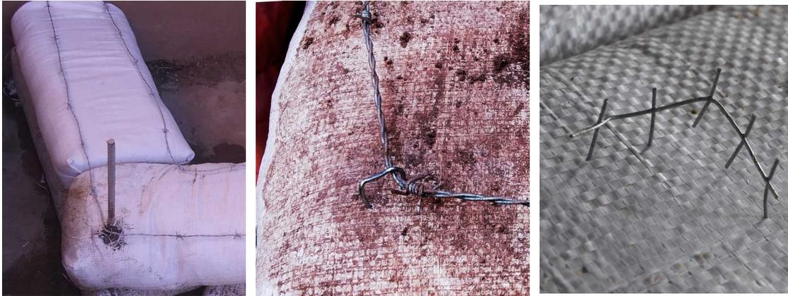
Figure 19 Hold barbed wire in place (left to right): a- Wrap around a vertical rebar; b- Tack wire at corners with an electrician's staple; d- Tack with pins cut from wire mesh.
