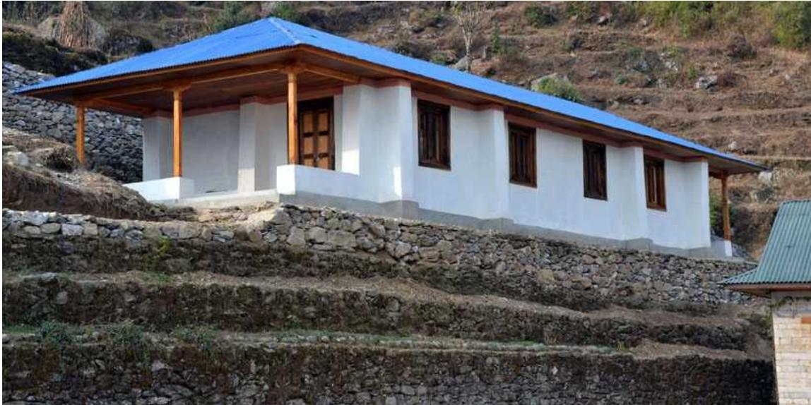
*Figure 3: Plastered School in Phuleli by Edge of Seven and Small World Nepal survived the 2015 earthquakes without damage despite earthbag construction with conventional techniques.*
