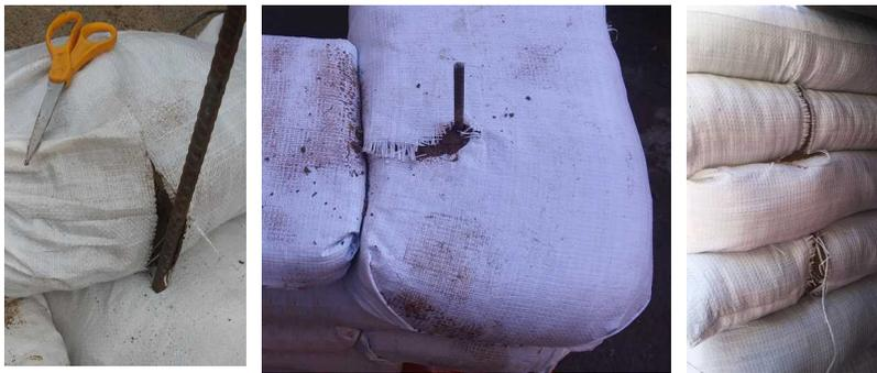
*Figure 29: Cut-bag construction (left to right): a- Cut tubes in place on the wall; b- Located at a protected inside corner; c- Alternating sides on a straight wall.*
