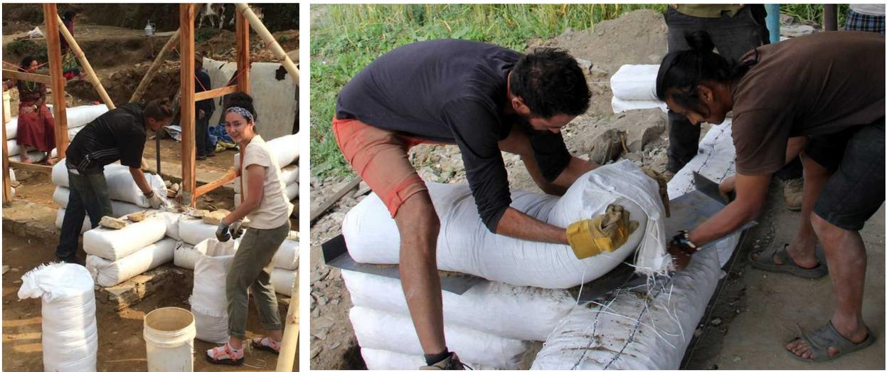
*Figure 18 Earthbag in Nepal (left to right): a- 150 mm (6") high tubes filled while containers are upright (T. Nillson used by permission); b- Adjusting a buttress tube on a wall (First Steps Himalaya used by permission).*
