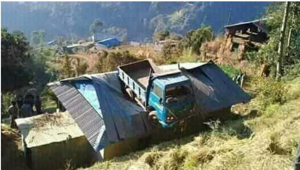
*Figure 6: Roof was damaged but not the earthbag walls by this truck accident (C. Ziegler, used by permission).*
