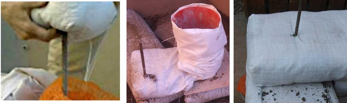
*Figure 27 Punched-bag construction (left to right): a- Cut the hole before filling, then slide a partly-filled tube end over a rebar; b- Continue filling the tube; c- Tamped punched-bag.*
