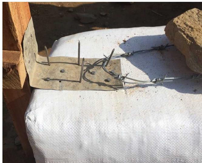
*Figure 4 Basic earthbag construction (left to right): a- Curved course edges with barbed wire on the flat course top; b- Velcro plate used to connect earthbag to wood elements (photo T. Nilsson used by permission).*
