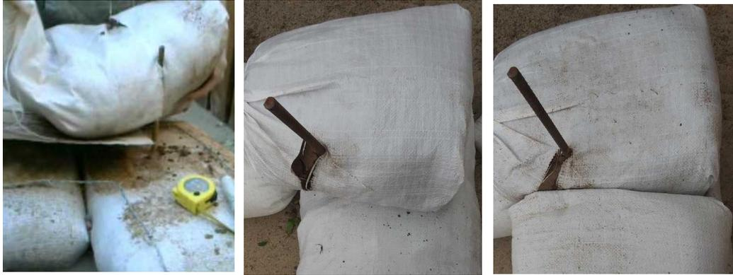
*Figure 30 Placing cut-bag tubes (left to right): a- Slide the tube on metal around the rebar; b- Enlarge the cut if needed; c- Place the adjacent tube end and then tamp.*
