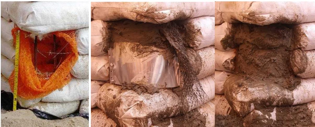
*Figure 34 Making the splice (left to right): a- Remove sandbag fabric, b- Place form and use mesh to fill the top, c- Concrete splice with mesh trimmed.*
