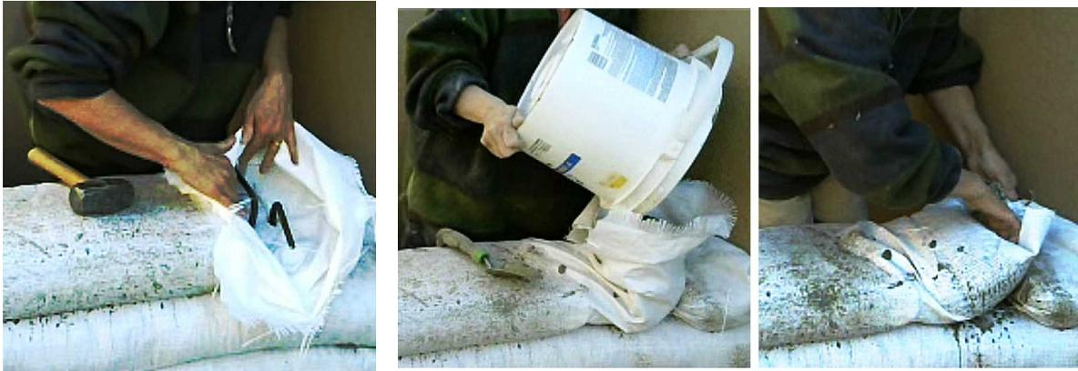
Figure 40: Splice on current course using tube as concrete form (left to right): a- Insert diagonal; b- Insert vertical; c- Both hooks fit within tube form on wall top.
