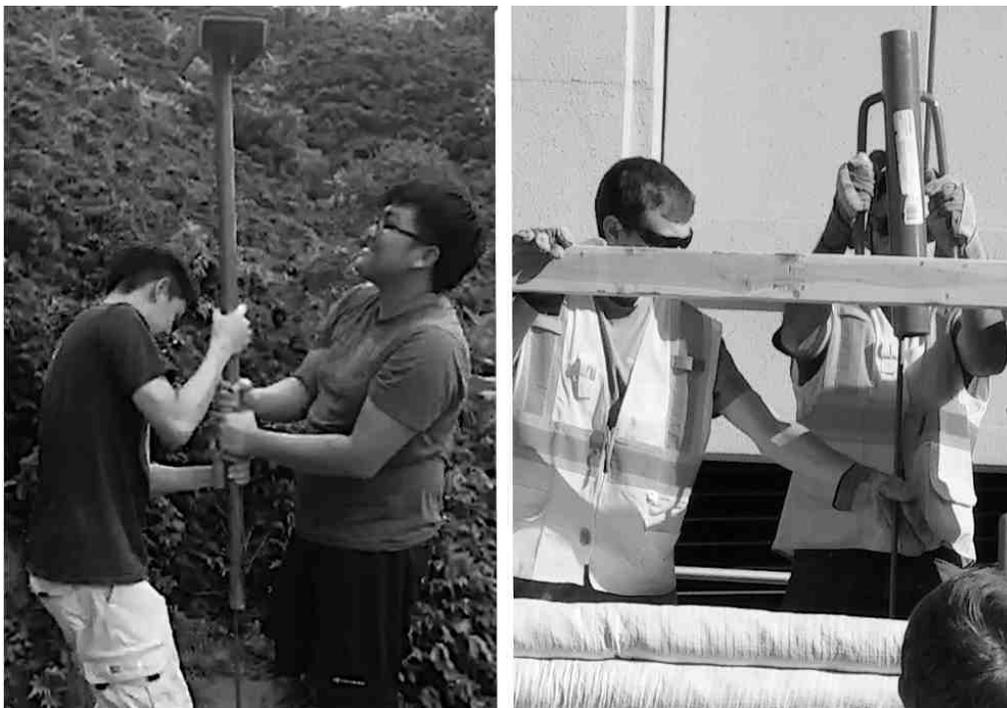
Figure 26 Tools to insert rebars (left to right): a- Steel welded on a pipe; b- Post driver tool.
