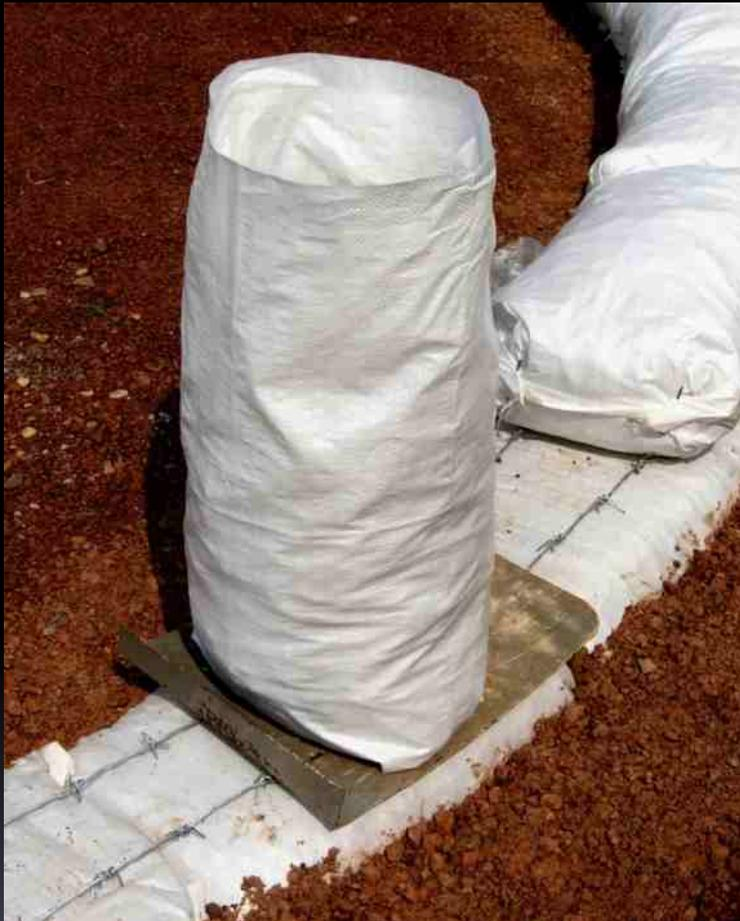
**Place bag or tube, lay down, then pull slider out**
