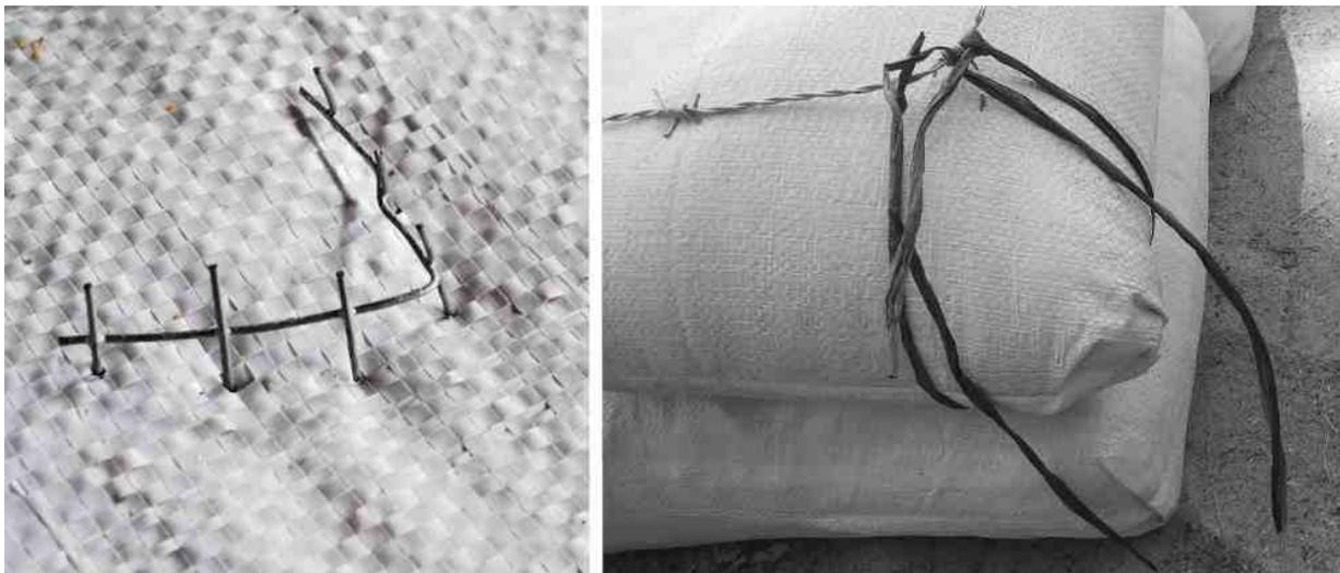
*Figure 32 Add strength where barbed wire turns corners (left to right): a- Pins cut from wire mesh and bent can pierce upper and lower courses, b- Tie wire from bends in barbed wire out both sides and up to the next course.*
