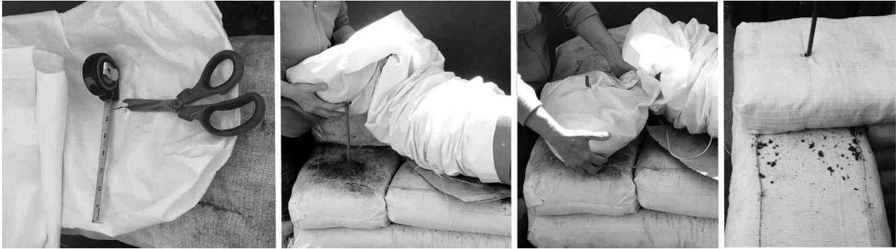
Figure 18 Punched-bag technique (left to right): a- Preparing holes near tube end; b- Slide partly-filled tube onto rebar; c- Slide top hole over rebar; d- Filled and tamped punched-bag tube.
