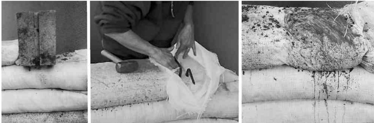
*Figure 21 Splice on current course using tube as concrete form (left to right): a- Tamp against block to form gap; b- Hooks of inserted rebars; c- Both hooks within concrete poured into tube wall top.*
