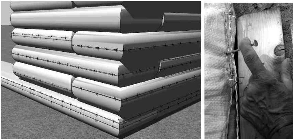
Figure 10 Wire binding (left to right): a- Bind around gravel bag courses; b- Pull both strands taut with a nail through wires at overlap.
