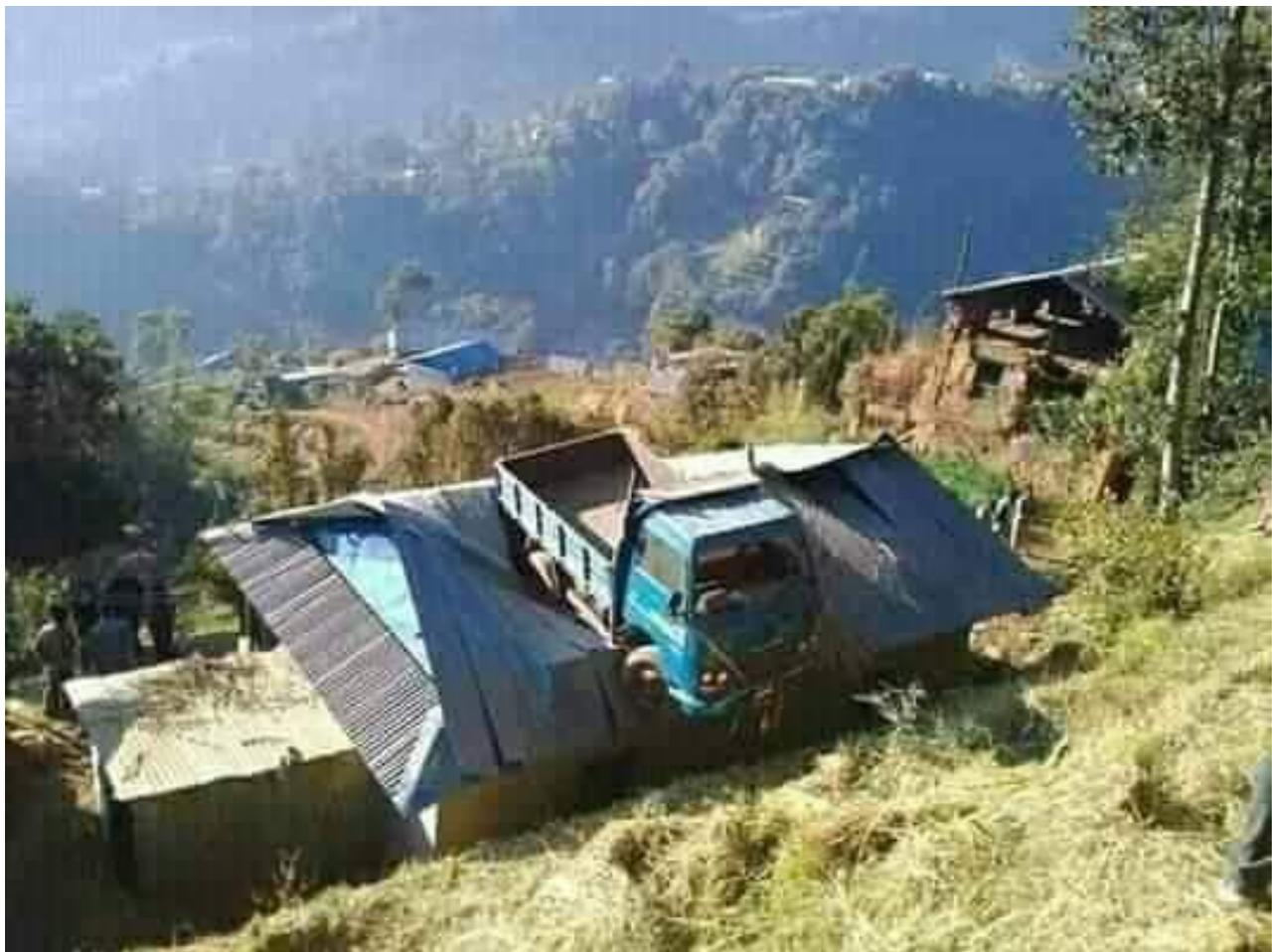
*Figure 3 Roof but not walls of earthbag building damaged by truck accident.*
