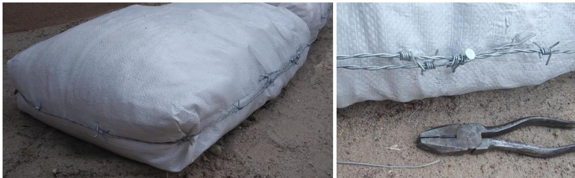
Figure 14 (left to right) Binding gravel bag courses: a- Wrap straight lengths; b- Attach securely.
