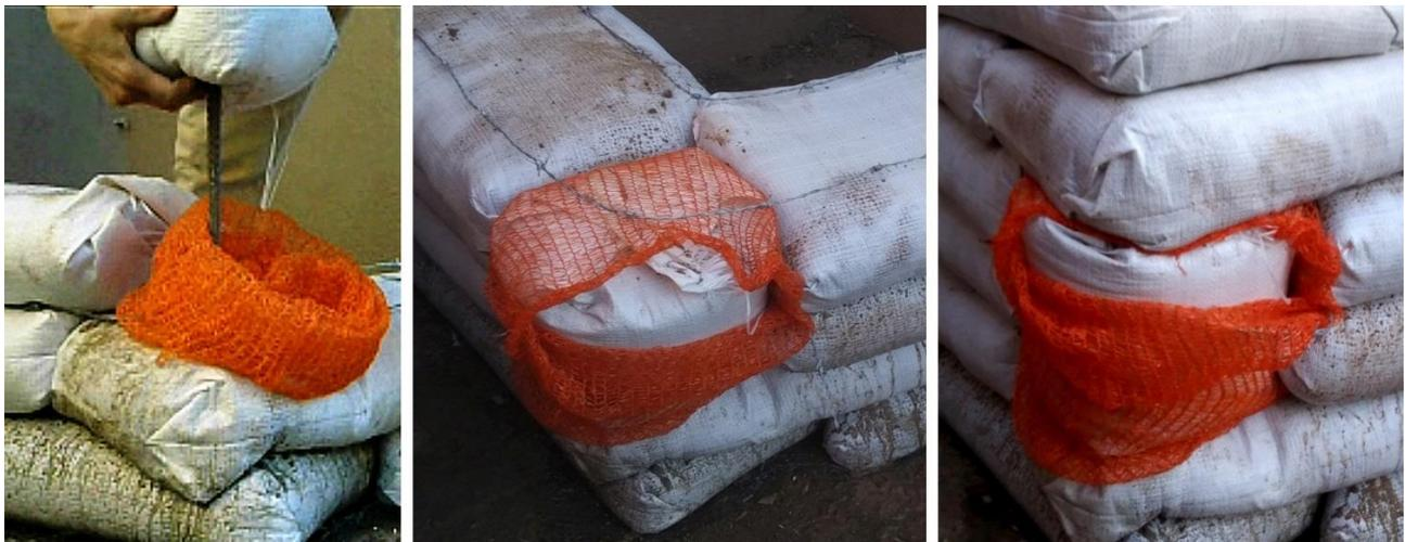
*Figure 29 An upright sandbag for a covered splice (left to right): a- Insert the sandbag into the mesh tube; b- Build courses next to the sandbag; c- Add courses above splice to final wall height.*
