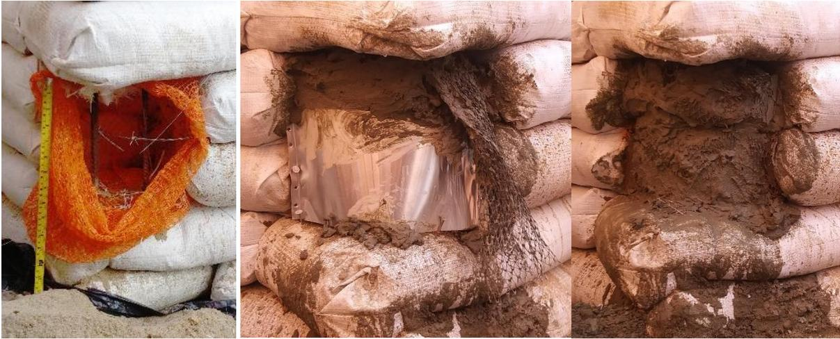
*Figure 30 Making the splice (left to right): a- Remove sandbag fabric, b- Place form and use mesh to fill the top, c- Concrete splice with mesh trimmed.*
