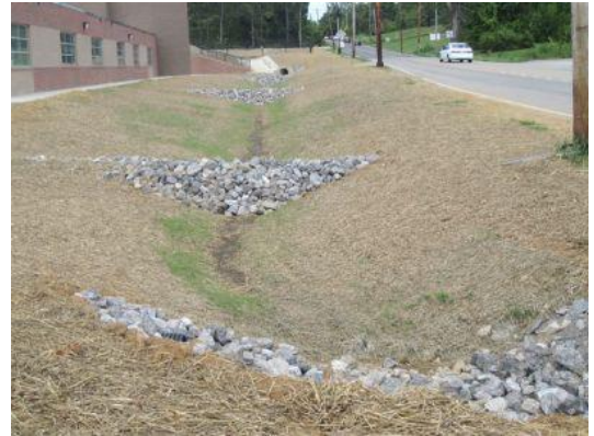
Image above: Erosion control checkdams 4 .
