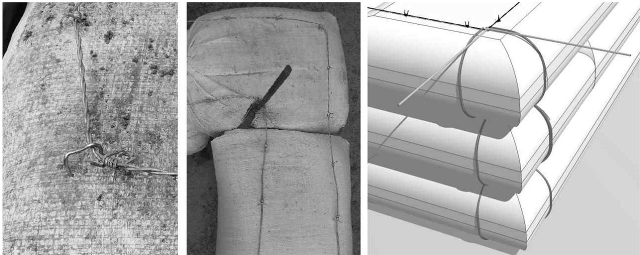
Figure 3 Barbed wire held taut by (left to right): a- electrician's staple; b- rebar; c- cord ties at corner.
