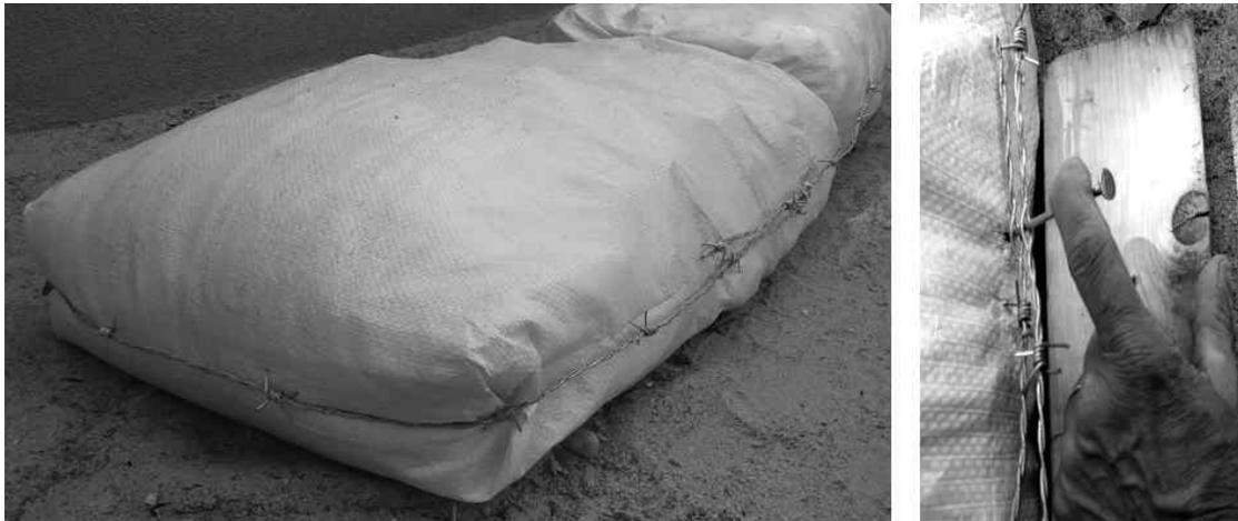
Figure 4 (left to right): Binding gravel bag courses: a- Wrap straight lengths; b- Attach securely.
