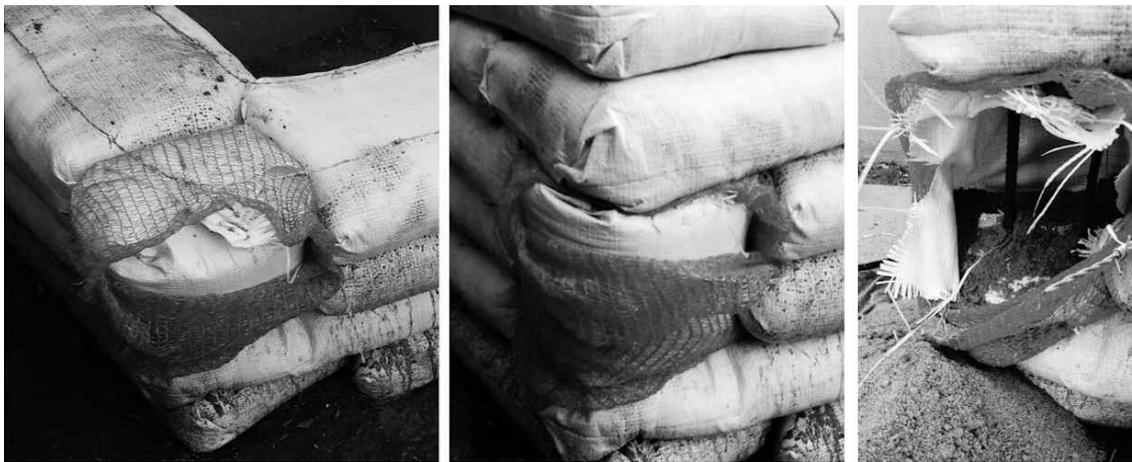
*Figure 13 Covered splice (left to right): a- target sandbag placed in mesh; b- building above the target bag; c- remove fabric and sand from target bag to create space for concrete.*
