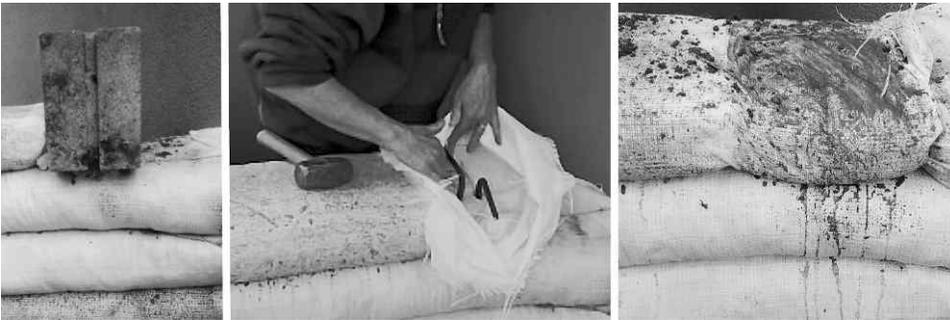
Figure 11 Open splice on top of a course (left to right): a- Tamp end of course at splice area; b- Insert rebars and turn hooks to fit; c- Pour concrete to embed steel into tube on top of course.
