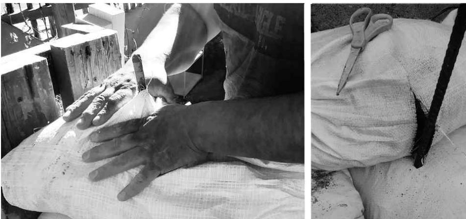
Figure 8 Embed steel by (left to right): a- punching bags; b- cutting tubes to fit around rebar.
