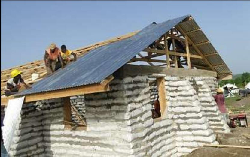
Use collar-ties or trusses so weight doesn't push wall tops outward
