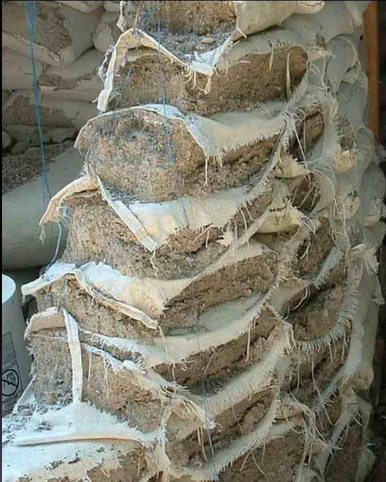
**Bags keep earth inside walls if stressed by quakes or vehicle damage.**
