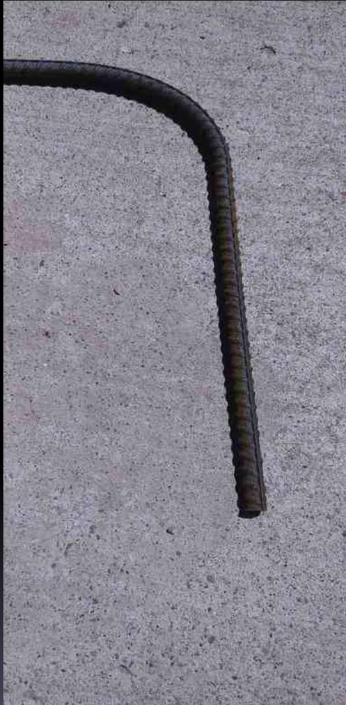
To embed 10" (250 mm) of rebar in a concrete bond beam, bend the top  $>90^\circ$  before inserting
