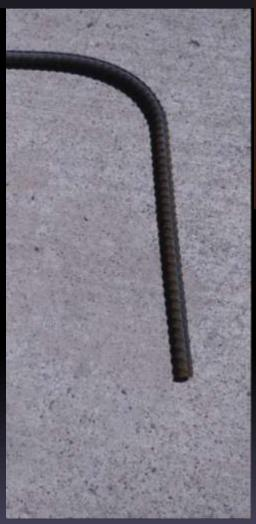
To embed 10" (250 mm) of rebar in a concrete bond beam, bend the top >90° before inserting
