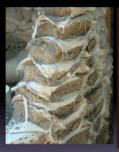
Bags keep earth inside walls if stressed by quakes or vehicle damage.
