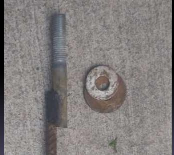
For a wood bond beam, weld a bolt on top
