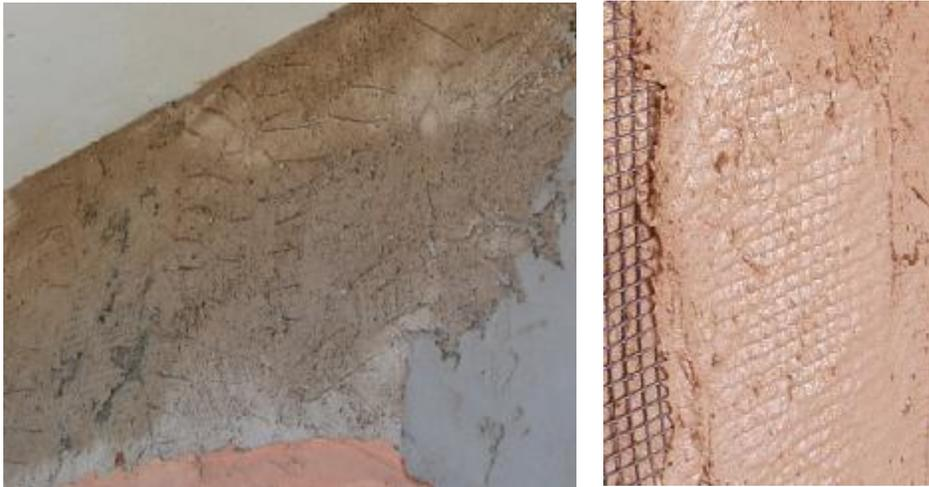
The gray layer shown at left is exterior earth plaster under a deep overhang in a very dry climate. It is also on the protected side of the buildings (not hit by storm winds).
