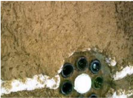
But always leave texture so the next layer of plaster will adhere. Poke finger holes or scratch the plaster before each layer dries.
