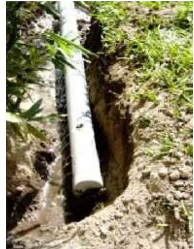
A cheaper system is to make underground water outlets from plastic buckets, clay flower pots, stones, bricks or blocks. Always try out your graywater system before you cover it up. The space in the pipe or buckets or under the blocks has to be big enough to hold all the water used until it soaks into the ground.
