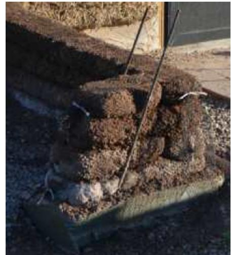
Before the top layer of the base wall, lay strong poly cord or wire across the wall. Then lay the top layer. Lay long cord on top of the last layer of base material. This will be used to snug the fiber tubes and keep them firm and level.
