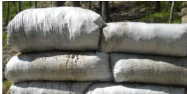
*Above: Damp, cohesive soil fill compacts when tamped*
