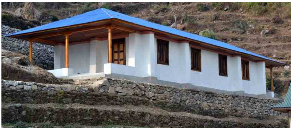
Figure 3: Plastered School in Phuleli by Edge of Seven and Small World Nepal survived the 2015 earthquakes without damage.
