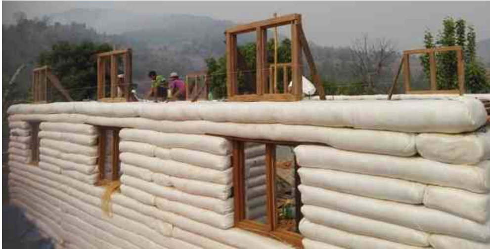
Figure 2: Earthbag building wall under construction in Nepal summer 2016.
