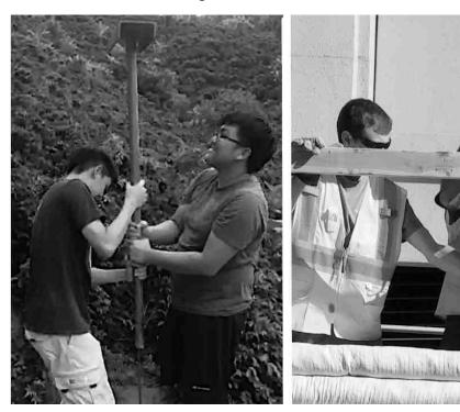
Figure 26 Tools to insert rebars (left to right): a- Steel welded on a pipe; b- Post driver tool.
