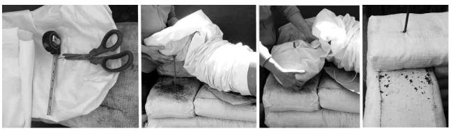
Figure 18 Punched-bag technique (left to right): a- Preparing holes near tube end; b- Slide partly-filled tube onto rebar; c- Slide top hole over rebar; d- Filled and tamped punched-bag tube.
