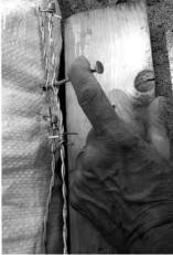
Figure 10 Wire binding (left to right): a- Bind around gravel bag courses; b- Pull both strands taut with a nail through wires at overlap.
