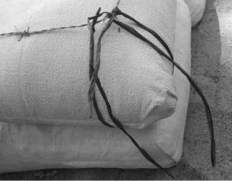
Figure 32 Add strength where barbed wire turns corners (left to right): a- Pins cut from wire mesh and bent can pierce upper and lower courses, b- Tie wire from bends in barbed wire out both sides and up to the next course.
