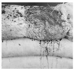
Figure 21 Splice on current course using tube as concrete form (left to right): a- Tamp against block to form gap; b- Hooks of inserted rebars; c- Both hooks within concrete poured into tube wall top.
