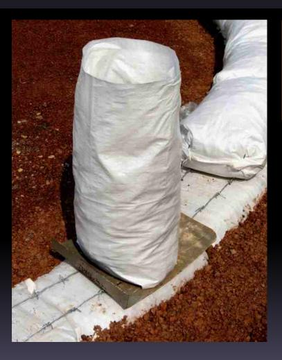
Place bag or tube, lay down, then pull slider out
