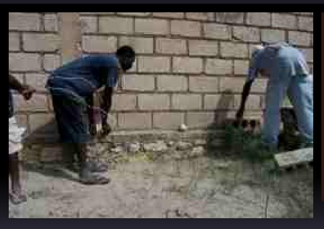
Mark the length on a wall, Stretch wire alongside, cut, place immediately
