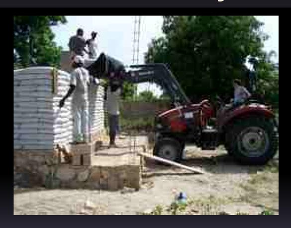
Use an auger or elevator if no loader is available
