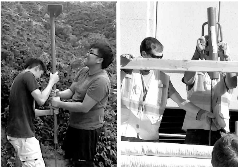
Figure 27 Tools to insert rebars (left to right): a- Steel welded on a pipe; b- Post driver tool.
