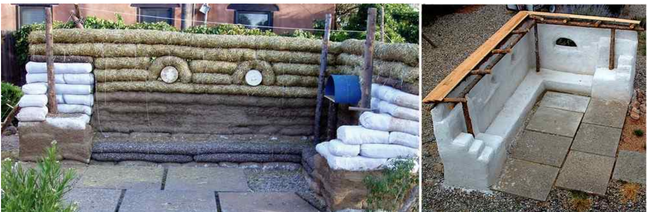
Figure 14: Left: Straw log bench wall attached to earthbag buttresses at each end. Right: Banco with lime plaster covering earthbag, gravel bag bench and straw logs.
