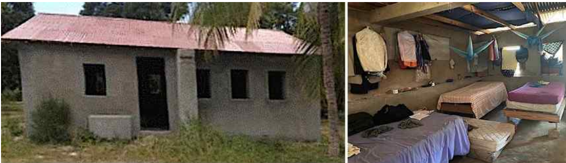
Figure 13 left: Haitian dormitories combined earthbag buttresses with reinforced concrete ceiling beams. Right: Current interior of the dormitory under intense use.
