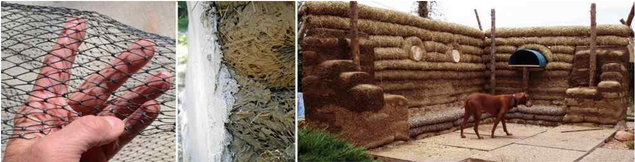
Figure 3 left: Wattle mesh. Center: Plaster skin on straw logs. Right: Straw log walls with formed windows.
