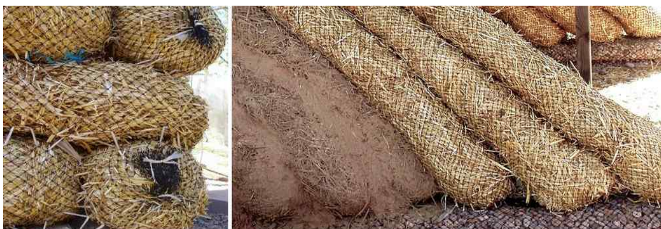
Figure 9 left: Sew all surfaces snugly at corner overlaps. Right: Partly soaked vault tubes sewn to mesh base.
