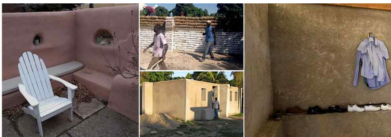
Figure 1- Straw log walls built in 2012/ 2013. Left: Banco with straw log walls in use today in Albuquerque, New Mexico. Center: Straw log dorm upper walls on earthbag base walls in northern Haiti before and after plaster. Right: Interior of straw log dormitory as currently in use shows stabilized plaster on straw walls above ledge of thicker earthbag base wall.
