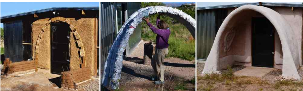
Figure 17 left: Panel of plastered straw wattle with arch form, behind thin earthbag base walls. Right: Stiff sewn tubes of wattle mesh filled with plastic trash. Right: Finished arch of trash tubes on earthen base wall.
