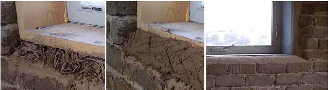
Figure 12 LSC to fill gaps- Left: Light straw-clay fills the gap under deep window framing of a thick veneer wall. Center: Leveling plaster of earth with little straw, textured to help finish plaster adhere well. Right: Finish plaster of earth smoothing edges of exposed adobe wall.
