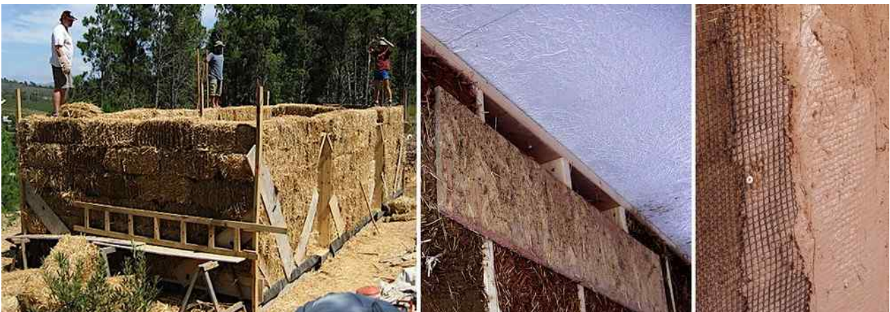
Figure 2 Left: Strawbale building by Philipp on Wikimedia Commons. Center: LSC infill in stud wall. Right: Earthen plaster embedding plastic mesh over straw-clay wall.
