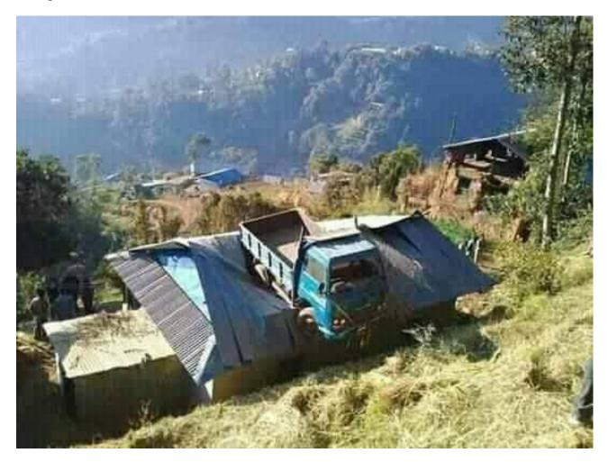
Figure 3 Roof but not walls of earthbag building damaged by truck accident.
