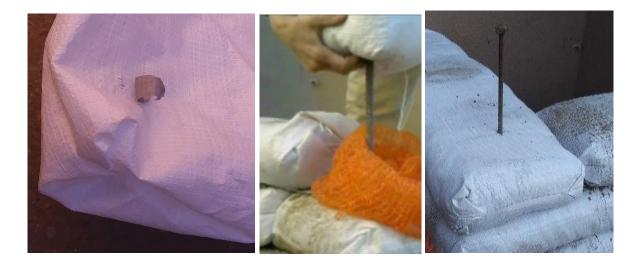
Figure 18 Punched-bag technique (left to right): a- Prepared hole near tube end; b- Slide a partlyfilled tube end down over a rebar; c- Filled and tamped punched-bag with no fabric gapping.
