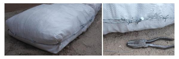
Figure 14 (left to right) Binding gravel bag courses: a- Wrap straight lengths; b- Attach securely.
