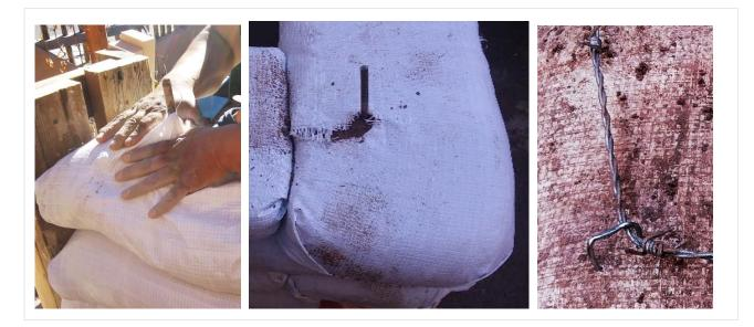
Figure 17 Techniques to embed steel (left to right): a- Punch bags onto anchored rebar; b- Cut tubes to form around rebar; c- Tack wire corners taut with an electrician's staple.
