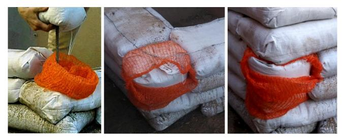
Figure 29 An upright sandbag for a covered splice (left to right): a- Insert the sandbag into the mesh tube; b- Build courses next to the sandbag; c- Add courses above splice to final wall height.
