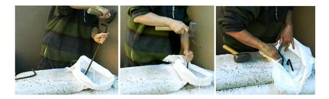
Figure 24 Splice on current course using tube as concrete form (left to right): a- Insert diagonal; b-Insert vertical; c- Both hooks fit within tube form on wall top.
