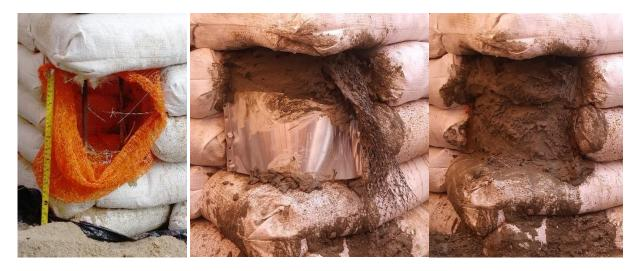
*Figure 30 Making the splice (left to right): a- Remove sandbag fabric, b- Place form and use mesh to fill the top, c- Concrete splice with mesh trimmed.*
