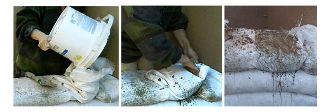
*Figure 25 Pour splice on current course (left to right): a- Add concrete inside tube over rebar hooks; b- Shake concrete in place and tuck bag end under; c- Finished splice level with course.*
