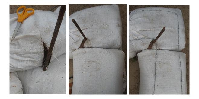
Figure 19 Cut-bag technique (left to right): a- Cut the tube next to the rebar; b- Slide the cut tube into position to surround the rebar; c- Running barbed wire past rebar.
