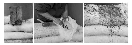
Figure 11 Open splice on top of a course (left to right): a- Tamp end of course at splice area; b-Insert rebars and turn hooks to fit; c- Pour concrete to embed steel into tube on top of course.
