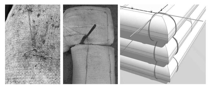
Figure 3 Barbed wire held taut by (left to right): a- electrician's staple; b- rebar; c- cord ties at corner.
