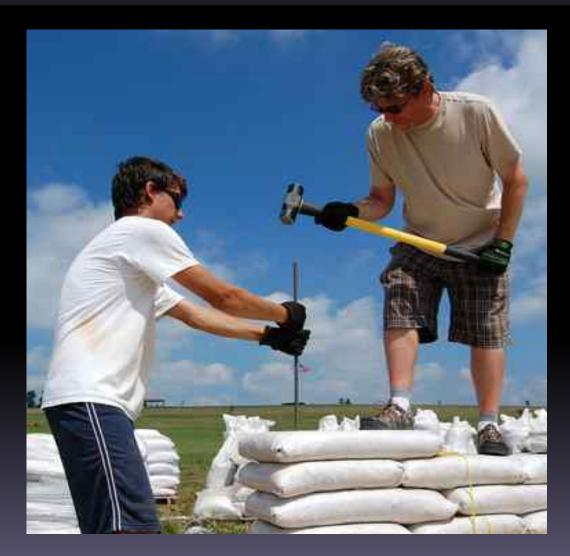
Hammer 5- 6' (1.5-1.8 m) lengths into damp walls
